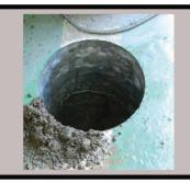
**STEP 4**Remove insert and clean hole of debris
